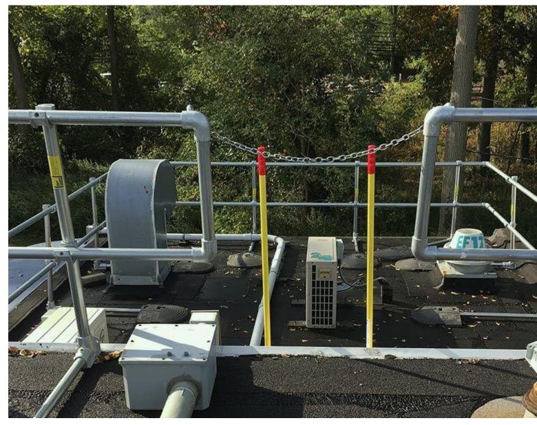
Please see an excerpt from a recently published story by *John Braun- CHST CSP* addressing the use of "Chains" as a means to prevent falls, through a fixed mounted ladder opening.
